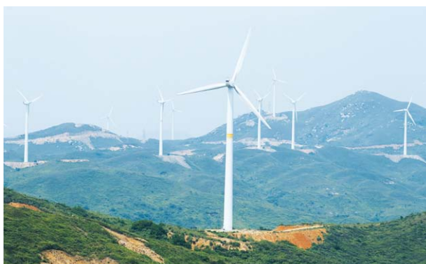
Wind turbines at the Chaonan Shalong Wind Project
