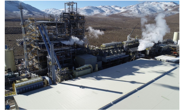
Fulcrum BioEnergy's Sierra BioFuels Plant in start-up operations, January 2022
